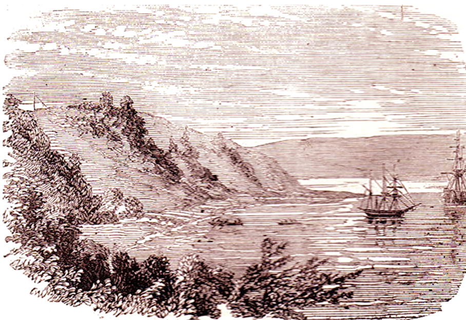
◀ Conveying the cable on shore near Varna.
